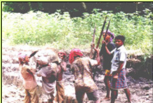
Young people working hard to build a village church.
